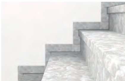
Joints on natural stone panels
