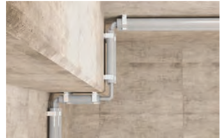
Fixing plastic insulating conduits
