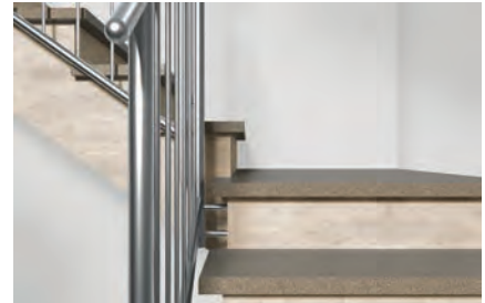
Stair treads on concrete stair stringers
