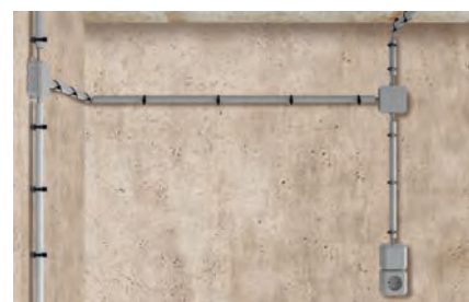
Flexible and rigid plastic pipes
