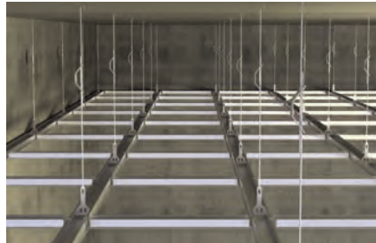
Suspended ceilings with Nonius hangers
