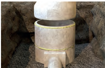
Sealing concrete manhole rings
