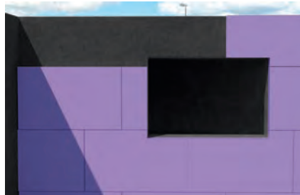
Bonding perimeter insulation boards
