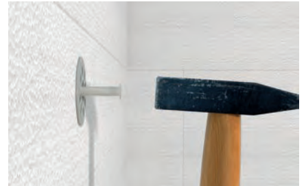
Setting the hammerset fixing on polystyrene rigid foam boards
