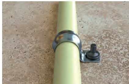
Fixing armoured conduits
