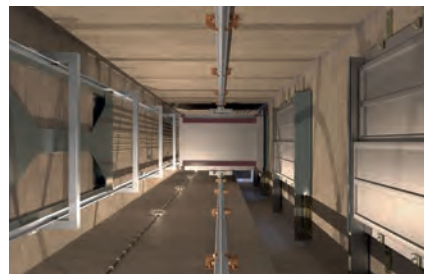
Guide rails for elevators
