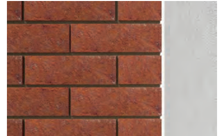
Joints between buildings
