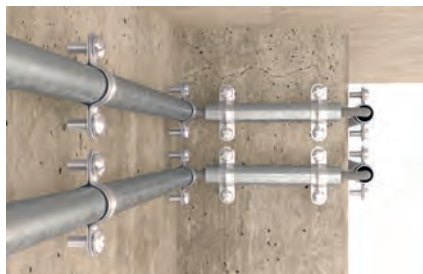
Fixing steel armoured conduits
