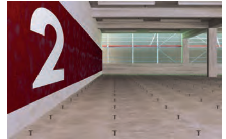
Reinforcement of ceilings
