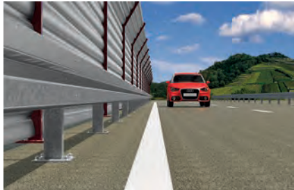
Crash barriers and sound insulation walls
